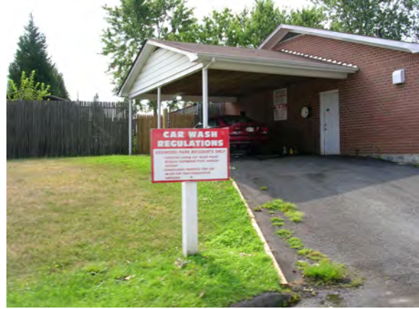
car wash where runoff goes to stormdrain in NSA-L-19
