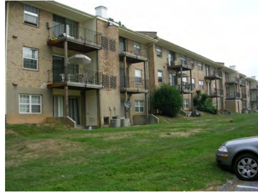
downslope disconnection opp. in NSA-L-21
