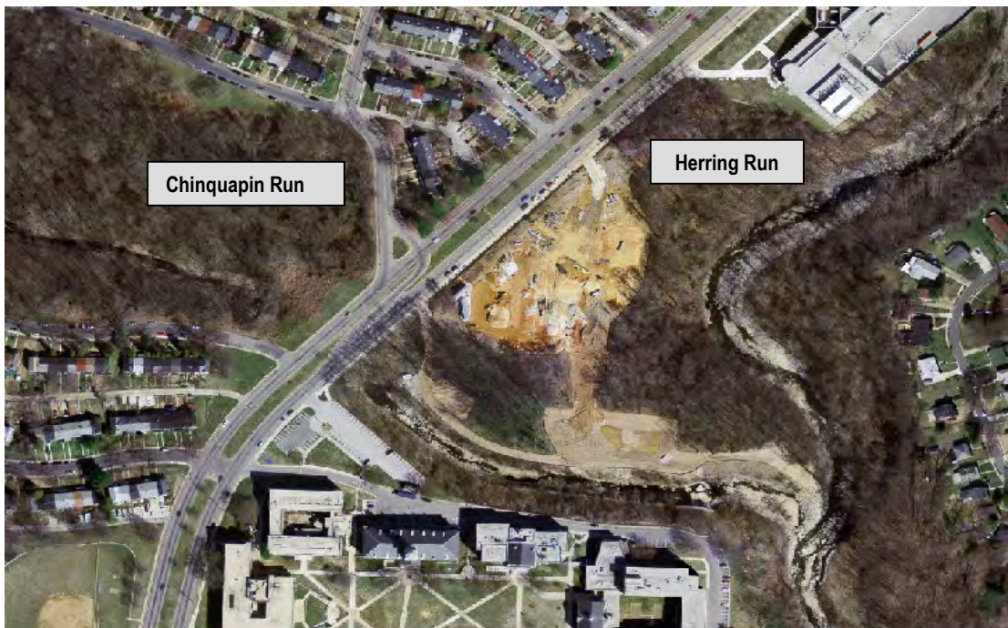
Morgan State construction project in Chinquapin Run buffer area where it joins Herring Run
