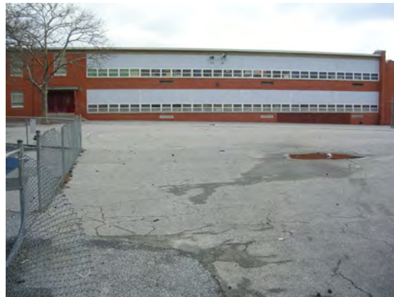
Impervious removal and good housekeeping at ISI-L-105
