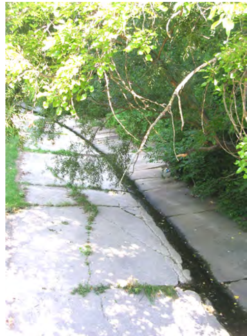
concrete channel in NSA-L-145
